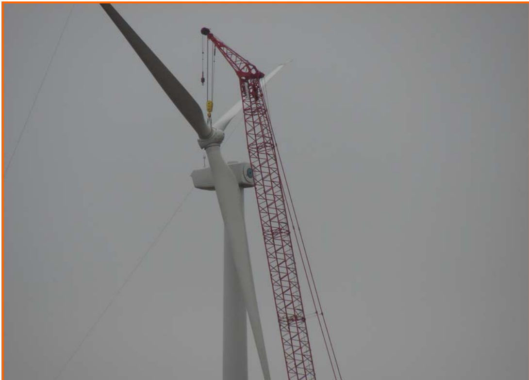
Putting on the blades and hub, notice the guy standing on the generator.
