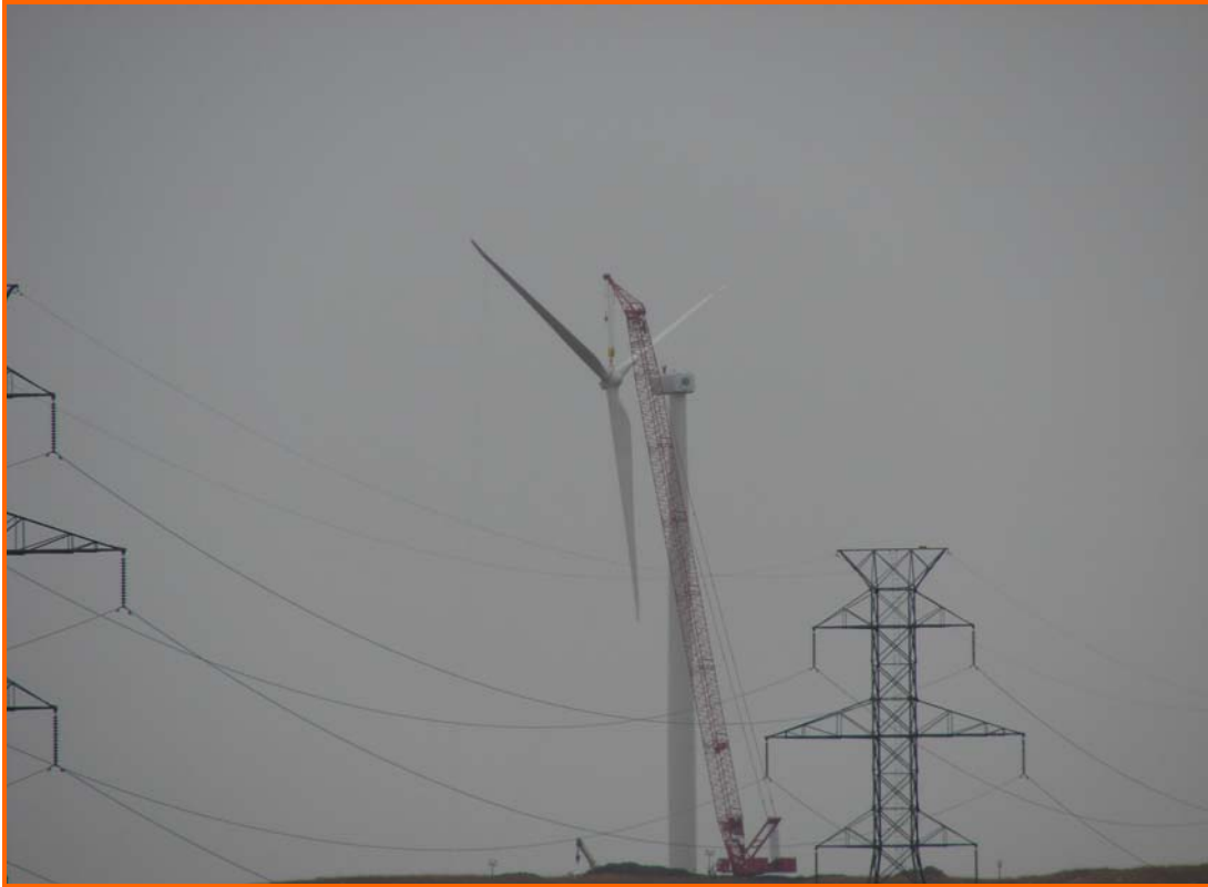
Putting on the blades and hub, notice the guy standing on the generator.
