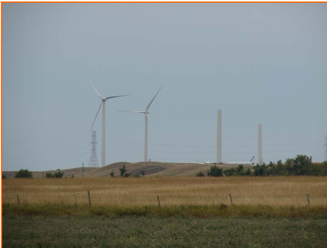
Some finished towers alongside some unfinished towers.
