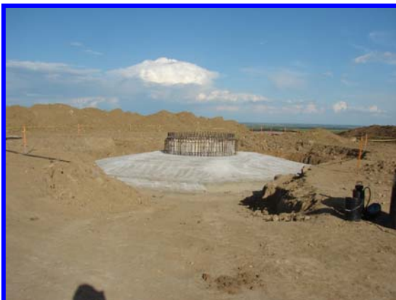
Finished footing, awaiting next phase of tower construction.
